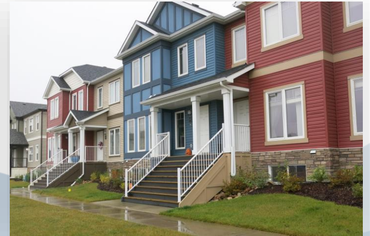
WINCHESTER ON PARK - 28 UNITS
